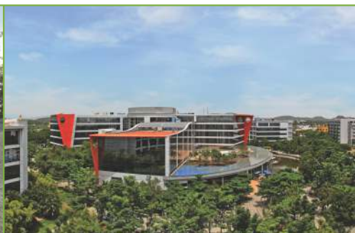
World cities - Integrated cities that improve the quality of life, living and livelihood for their occupants, and provide a stable infrastructure for organisations to invest in
