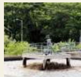
Reducing freshwater requirement through recycling
